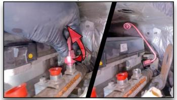
56. Loosen #6 Fuel Line, Rotate Out of Way
